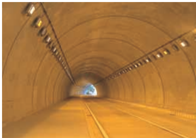
曇天時照明状況(1/2点灯) Lighting condition on cloudy days (Lighting of 1/2 capacity)
