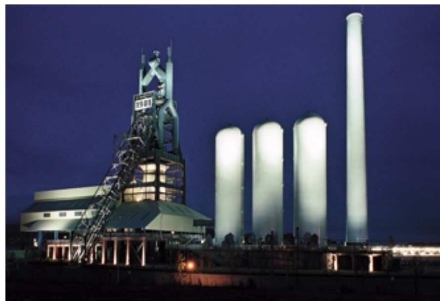
南東側景観 View of the south east side
