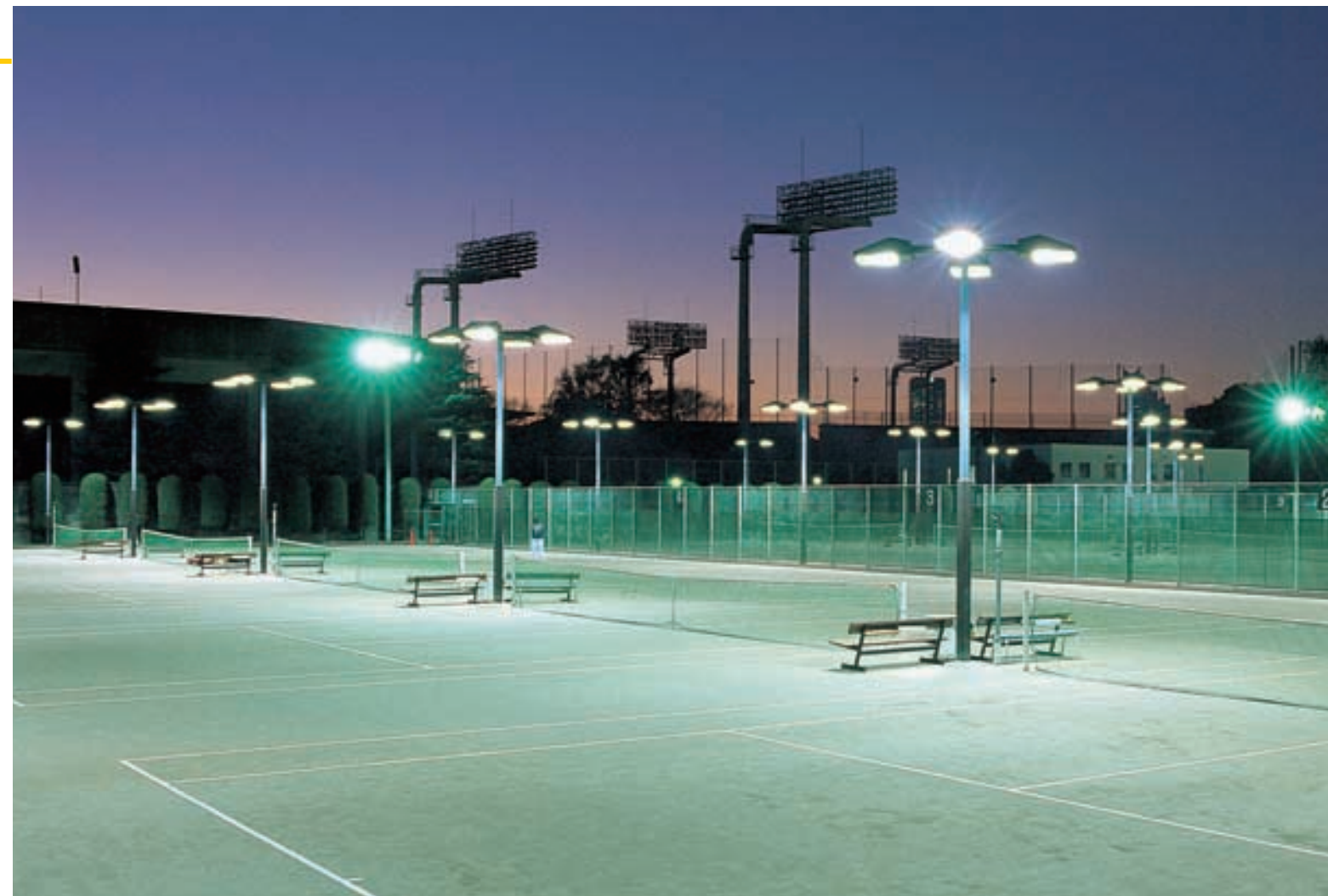
薄暮照明点灯時 Illumination at sun set
