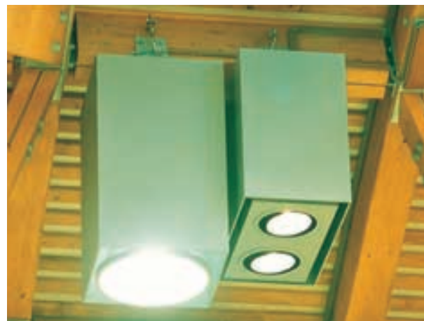
1階パークゾーン電動昇降式照明器具 Lighting apparatuses with electric-lift are installed for the indoor park-zone on 1st floor
