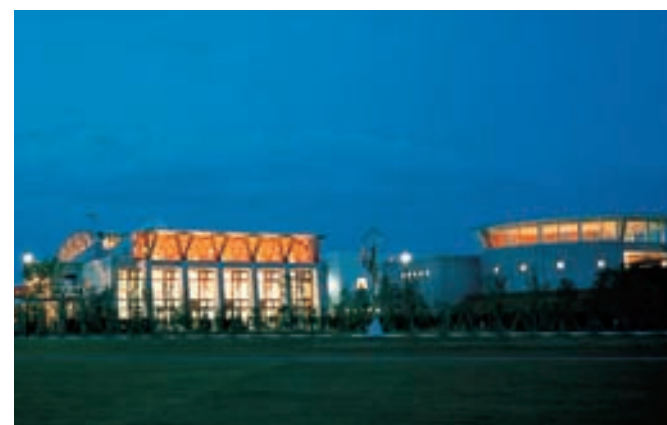
薄暮時の外観全景 Entire view of the structure in the evening
